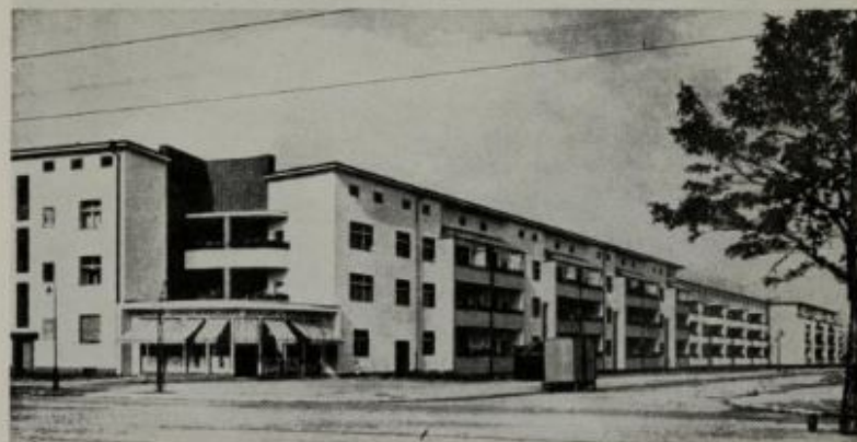
114. Bruno Taut. 'Gehag' housing, Berlin-Britz, 1927: low cost mass-housing of the sort that established the unique character and standing of the Berlin school.
