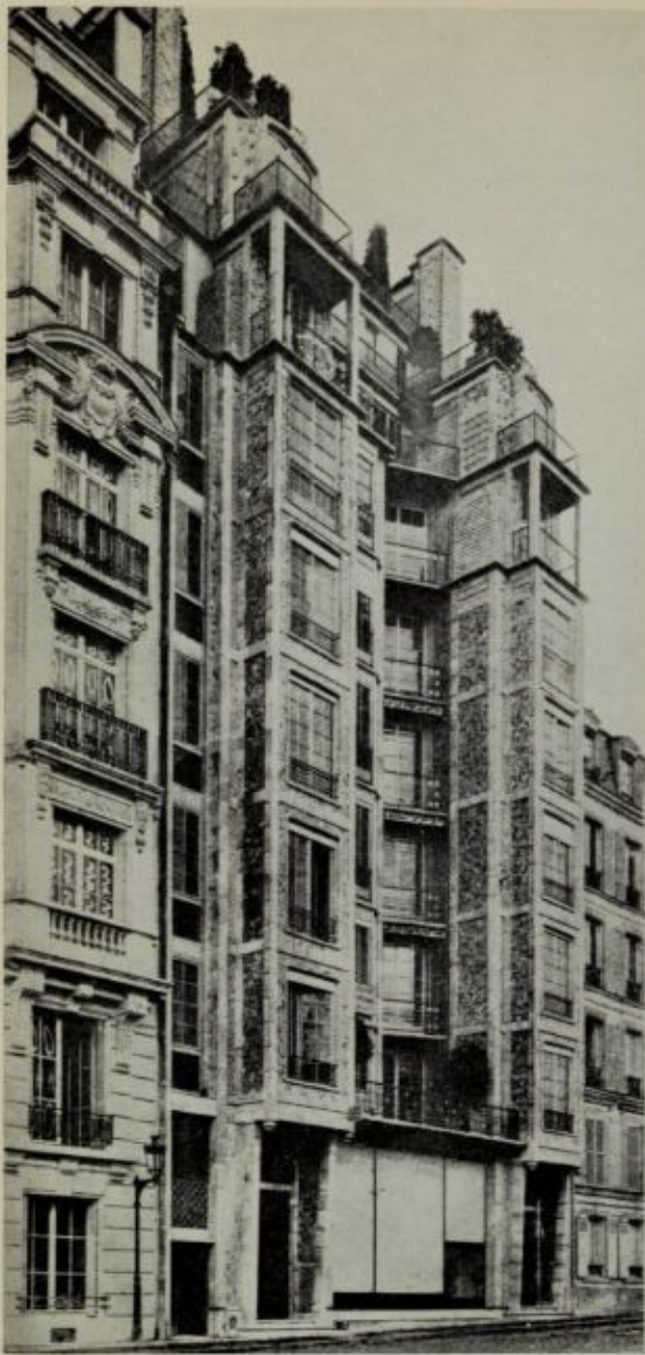
12. Auguste Perret. Apartment block in the Rue Franklin, Paris, 1903; a pioneer use of reinforced concrete in domestic work, notable for the ingenuity of its hollow U-fronted plan and the clear exhibition of its frame construction, although both structural and infill materials are clad in ceramic tiling.
