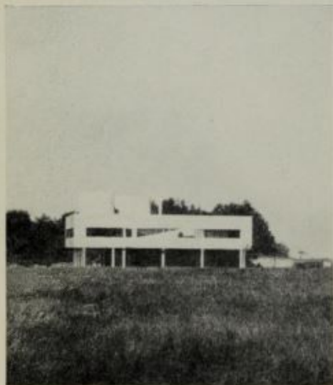
131, 132, 133. Le Corbusier and Pierre Jeanneret. Les Heures Claires , Poissy-sur-Seine, 1928–1930: the summation of the Latin stream in the International style—a post-Futurist villa, planned around a central ramp, raised on stilts for vehicle circulation, and set down, a pure aesthetic object, in an abstract landscape.
