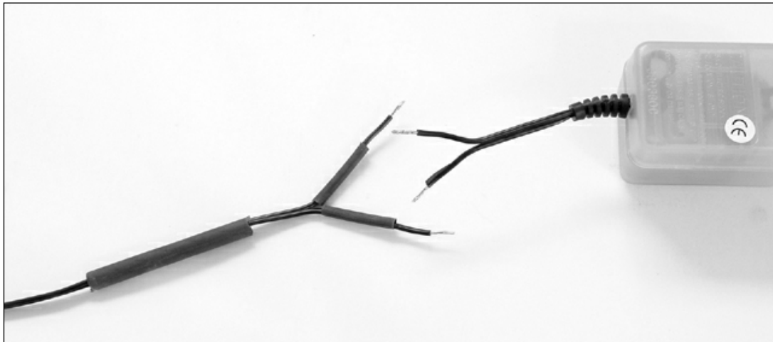
Figure 6.43 Successful Preparation of the Wires
